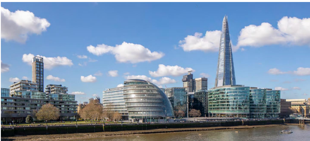
Existing building, taken from Tower Bridge and Existing:
