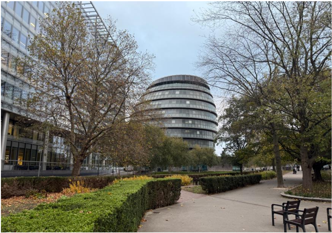
View of south elevation from Potters Field Park
